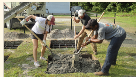
Project H staff and students (at construction site)
